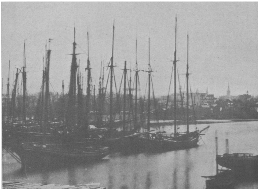
Courtesy Canadian Pacific Sealing schooners at anchor in harbor of St. John, New Brunswick
